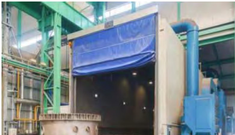
喷砂房 Blasting Room
